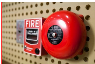
Fire Detection System
