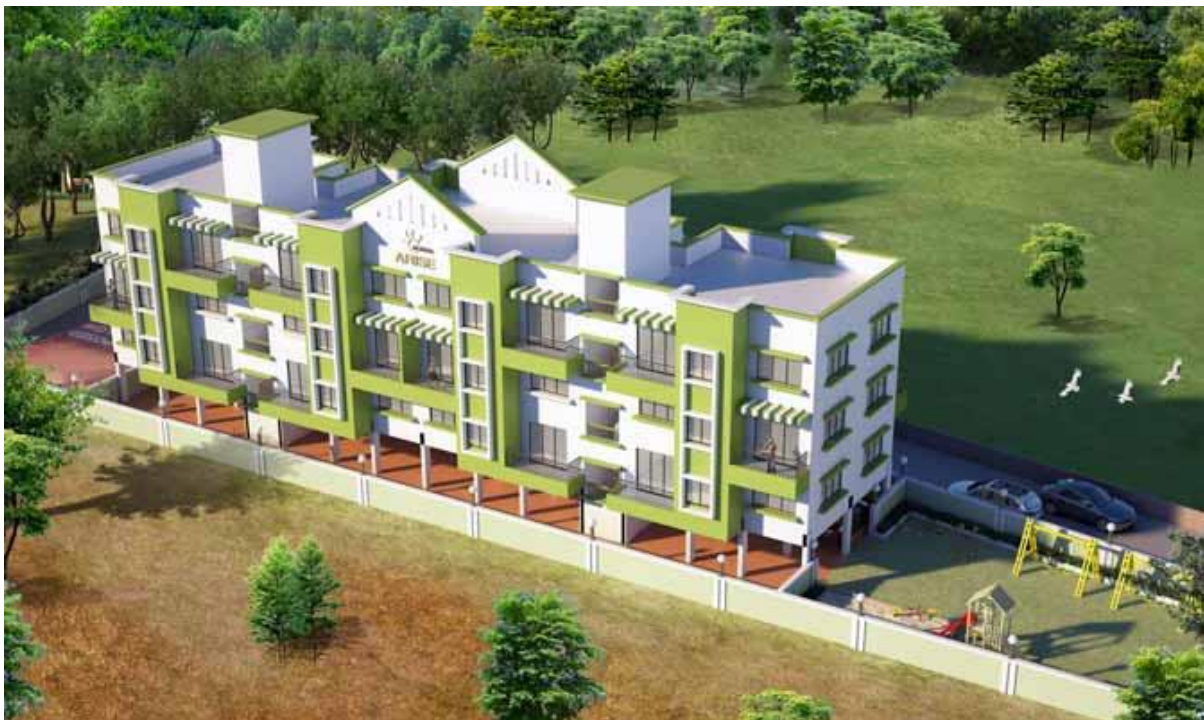
Project Name: Alisha Arise | Built Up Area: 16,000 sq.ft | Location: Guhagar
