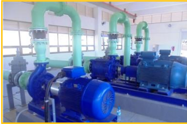
Water Supply, Pumping, Piping and Distribution
