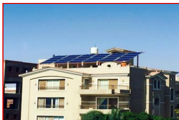
Solar Hot Water System
